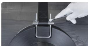
**b. Pre-tighten the branch using the mounting belt (black) and then tighten the mounting screws with a flat wrench 13 to fasten the saddle to the pipe**
